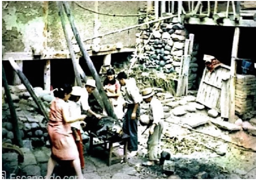
Fig. 4. Image of the construction technology applied. Source: Project report
