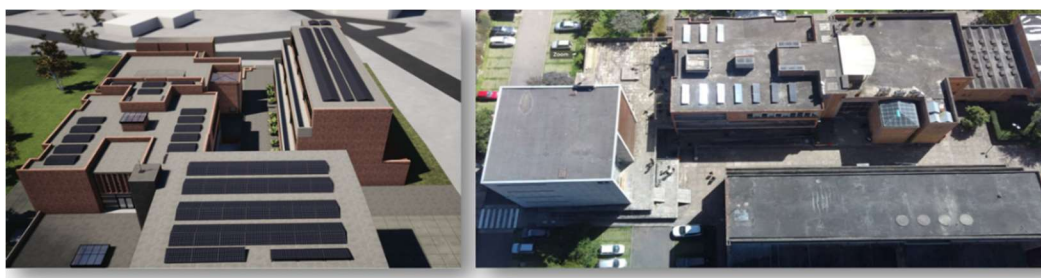
Fig. 6. Facultad de Arquitectura of the Universidad de Cuenca with projected total installation and in the right a 10 % of the solar plates installed in first instance. (Source Authors).
