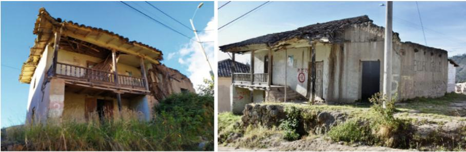
**Fig. 2. a-b.** State of deterioration of the “Lara-Espinoza” house before its intervention. Source: 2a: Achig, 2019. 2b: Astudillo, 2010
