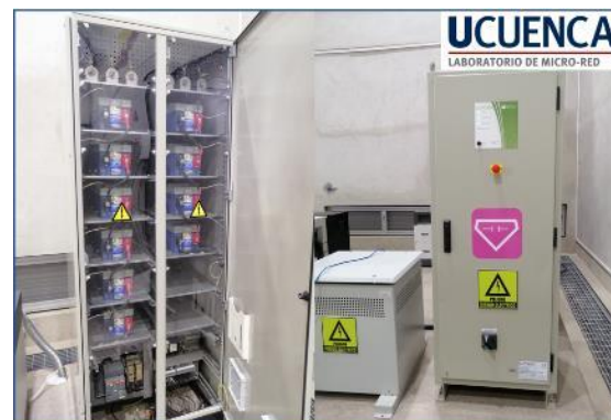
Figure A2. SC-ESS from the micro-grid laboratory: bank of supercapacitors (left), cabinet containing the power electronics converter (right).
