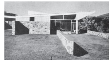
Figura 8. Casa Robinson, Williamstown, Massachusetts, 1946.
