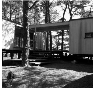
1963, Wise Cottage House, Wellfleet.
