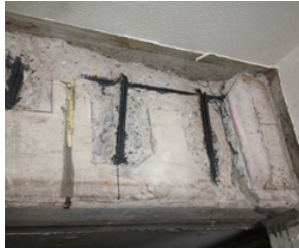
Figura 38. Descantilladura (waterproofing Brisbane)
