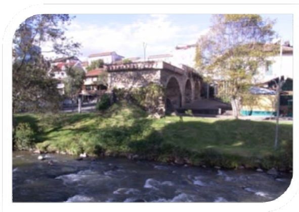
The Broken Bridge
