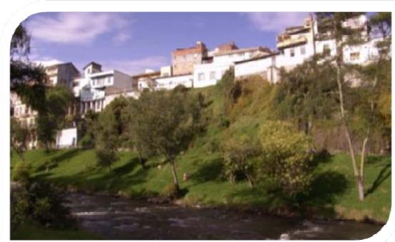
“El Barranco” of the Tomebamba River
