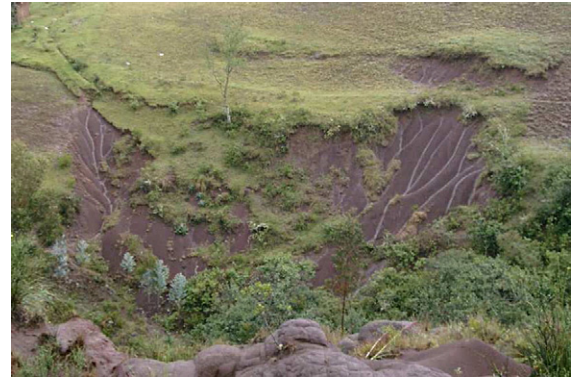
Fig. 6. Argillaceous rocks, highly susceptible to water erosion (Vegaspamba catchment).
