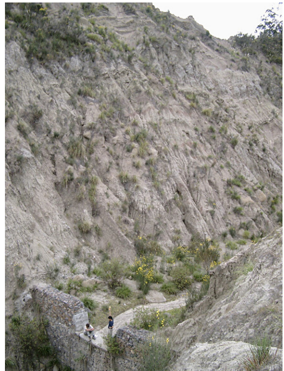
Fig. 2. Checkdams constructed in ephemeral stream channels to reduce the stream power (Caldera catchment). The mean annual sediment yield of this catchment of 1.48 \text{ km}^2 is the highest value that was measured in this region, and approximates 15,100 \text{ Mg km}^2 \text{ year}^{-1} .
