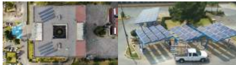
Fig. 2. SPV electricity generation system installed at CIC-IPN.
