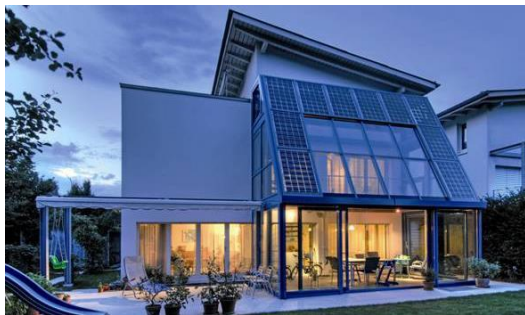
Figura 2.13: Building Integrated Photovoltaics – BIPV Fuente: Bureau, 2016
