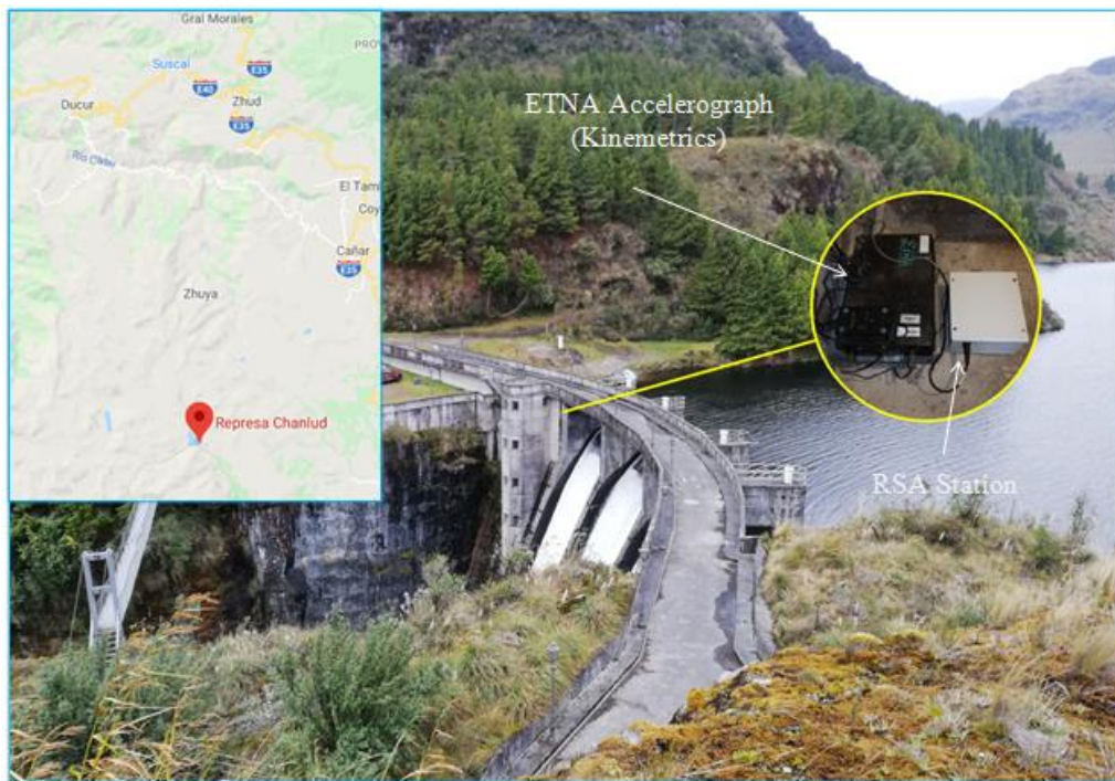
Fig. 8 Ubication of the accelerographs on the Chanlud hydroelectric dam
