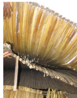
Figure 5. Roof layers (Hidalgo, 2007).
