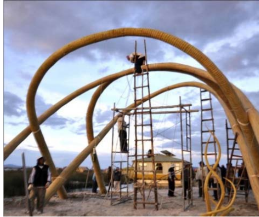
Figure 10. Totora Project, Community house structure. (PUCP & SAdBK, 2010).
