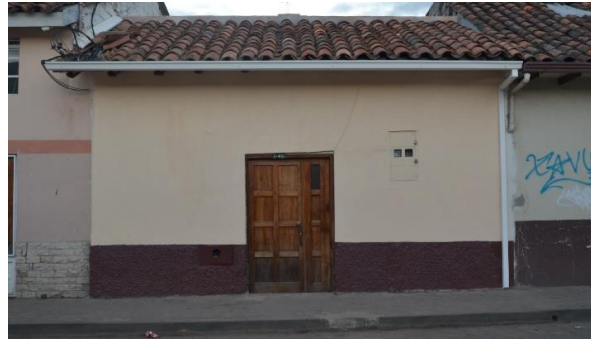
Figure 6. After the Herrerías Maintenance Campaign Source: City Preservation Management project.
