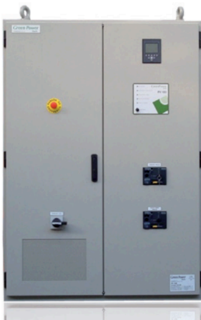
Figura 3-12 Inversor GPTech PV15
