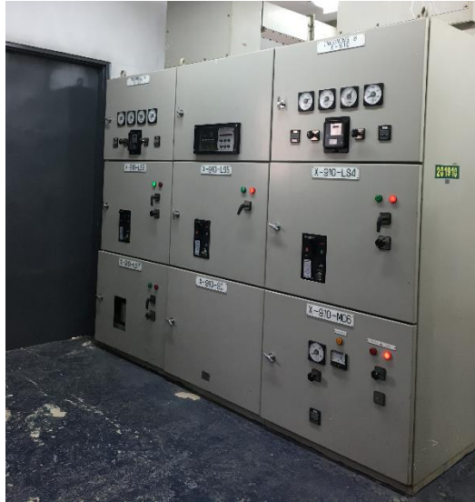
Figura 3.13.- Barra X-910, 480 V.
