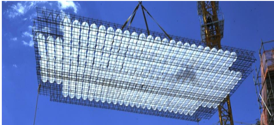
Figura 2.11 Losas Bubble deck (Reinforcement modules). [4]
